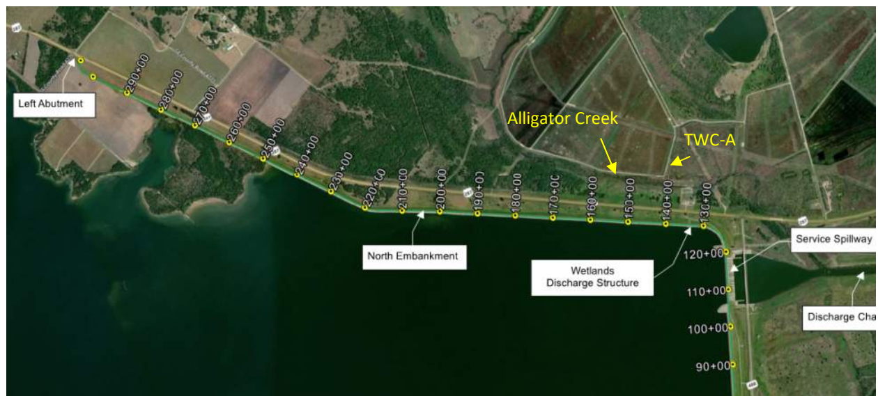
Figure 1: Overview of Richland Chambers – North Embankment
