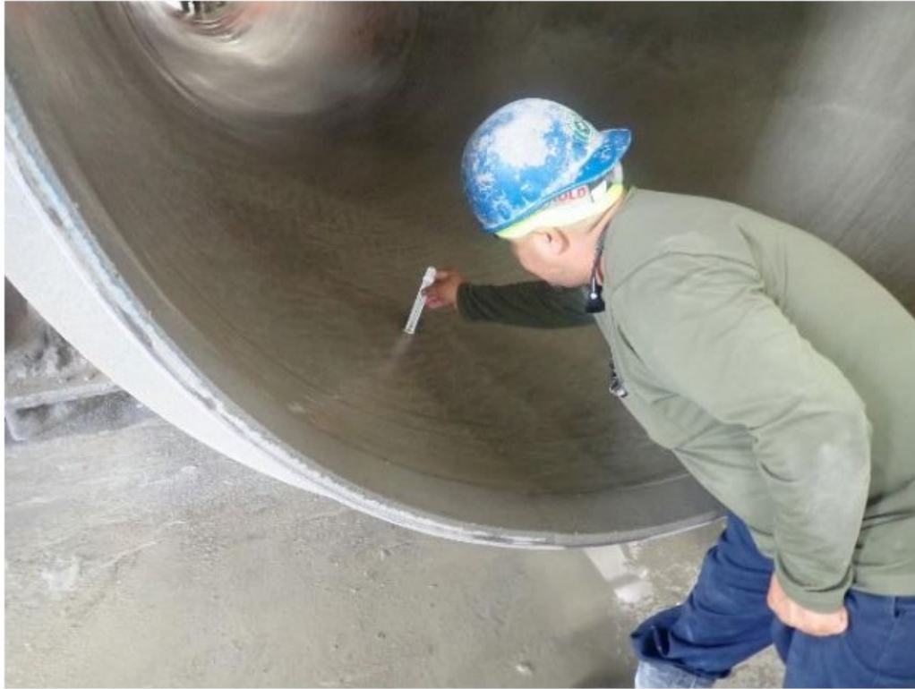
Cement Mortar Lining (CML) Thickness
