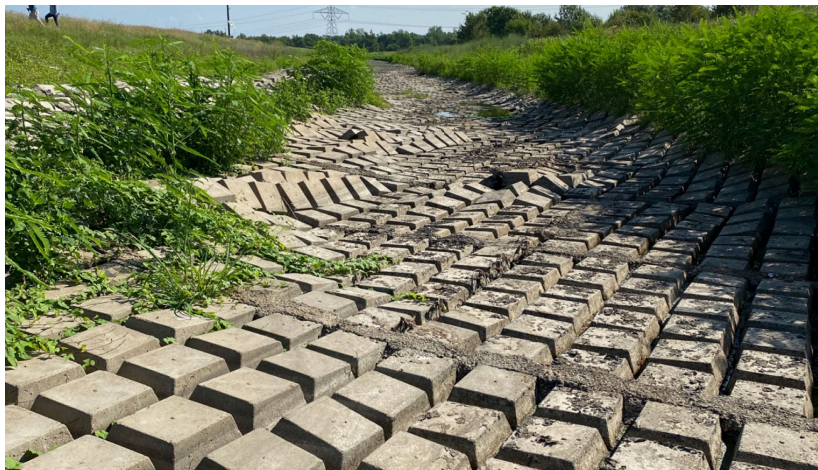
Localized uplift and buckling of articulated concrete blocks
