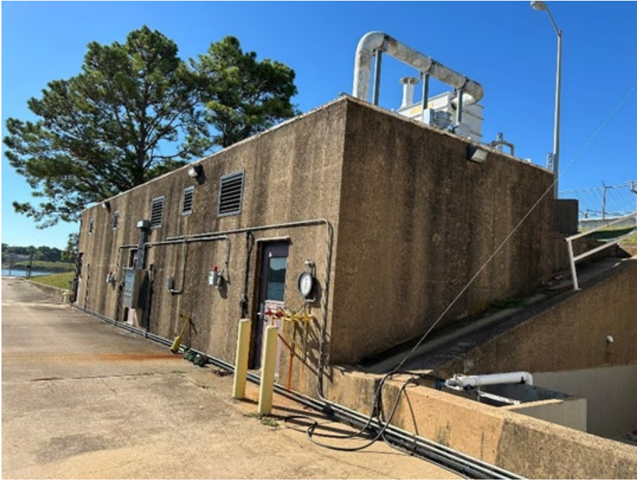
Chlorine Feed Room
