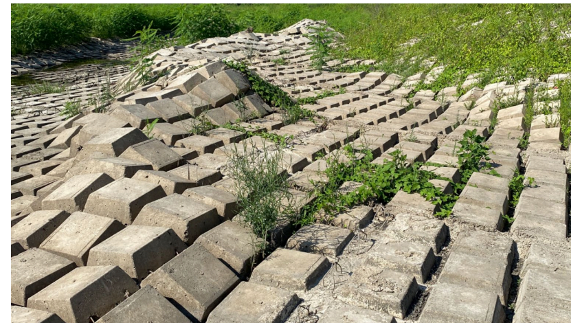
Localized uplift and buckling of articulated concrete blocks
