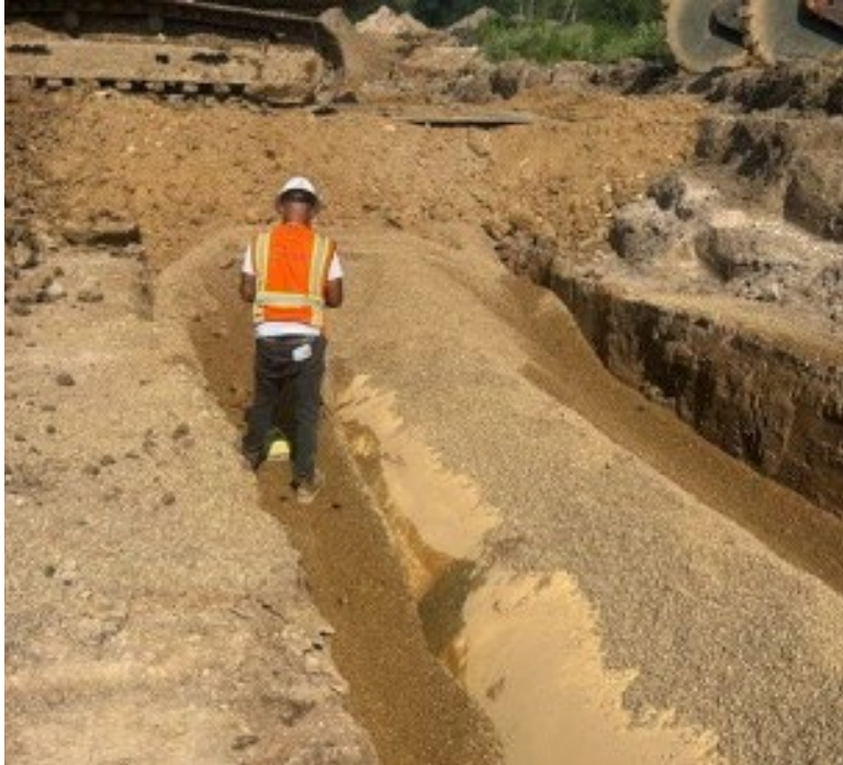
Soil Compaction Testing
