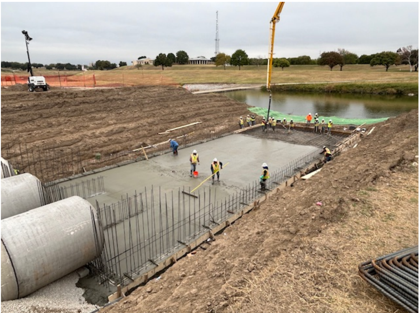
Central City Flood Control Project utility relocation work making way for bypass channel construction
