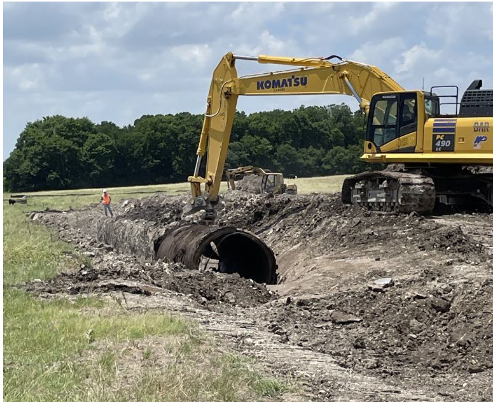
Cedar Creek Pipeline Phase 1 - removal of 72 inch, prestressed concrete cylinder pipe, June 2025
