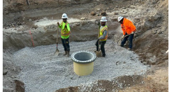
PL192A BOV Vault Installation
