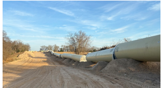
PL191A Pipe Strung Out on ROW
