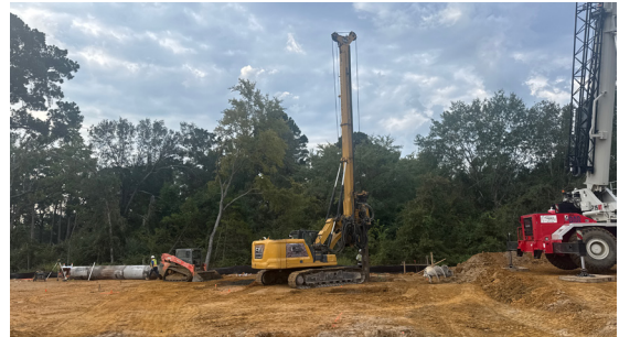
LP1HV Pier Drilling Activity
