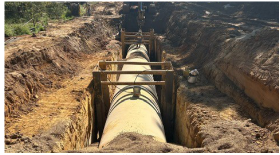
PL192A Pipelaying Installation
