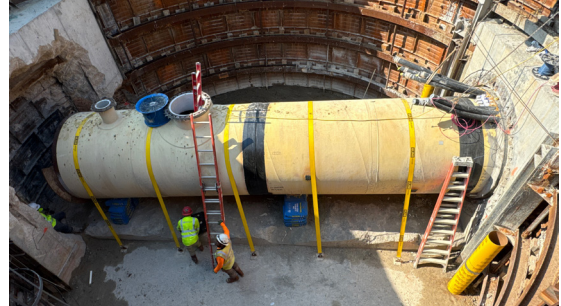
PL19TUN SH155 Launch Shaft Tie In Pipe
