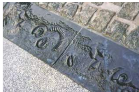
Hot Oil Dipped Iron Paver Inlay
