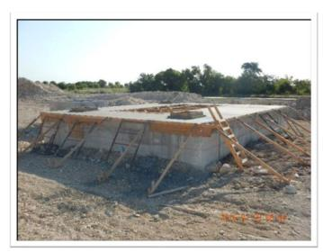
Armacon Type Gate Valve Enclosure
