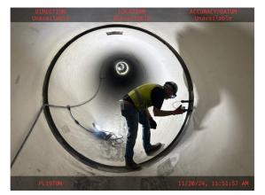
Joint Weld Magnetic Particle Testing
