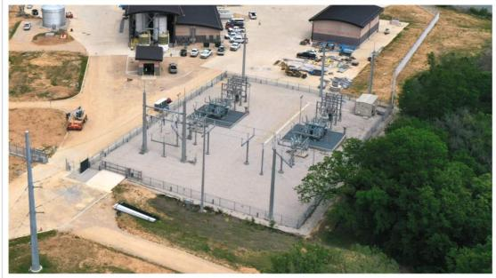
The Electric Substation takes in 138kV service from ONCOR and reduce to 5 kV service for drives, pump units and cooling systems.
