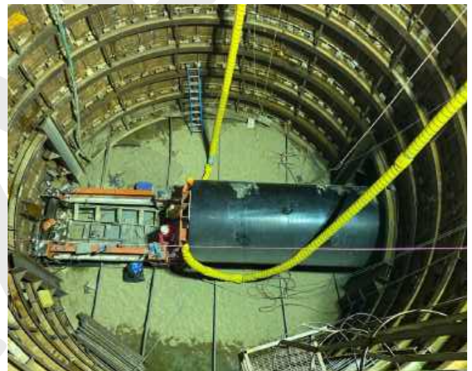
PL19TUN Pushing casing pipe into Stream A
