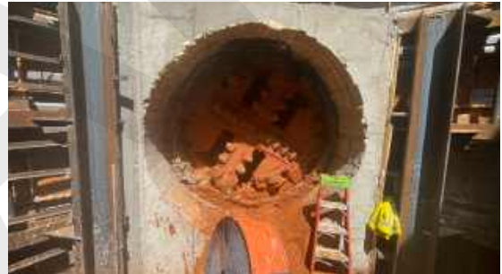
PL19TUN TBM Breakout into SH155 Retrieval Shaft
