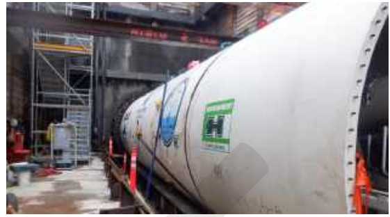
PL19TUN Cedar Creek Tunnel TBM Mining Operations
