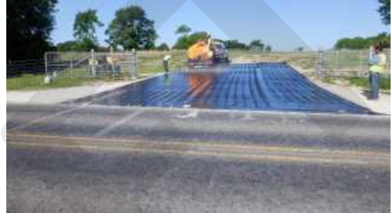
PL19TX Chipsealing Access Drive at Crossroads
