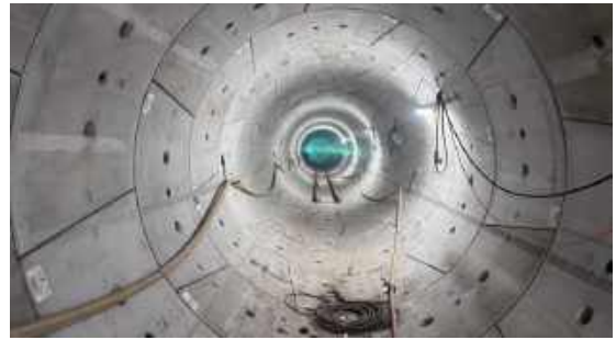
PL19TUN Completed Hollywood Lake Tunnel
