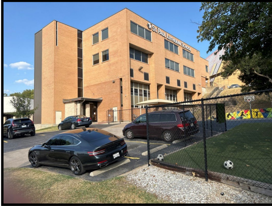
Figure 14 – Resource 89 – St. Paul Lutheran Church and School (Built 1969)
