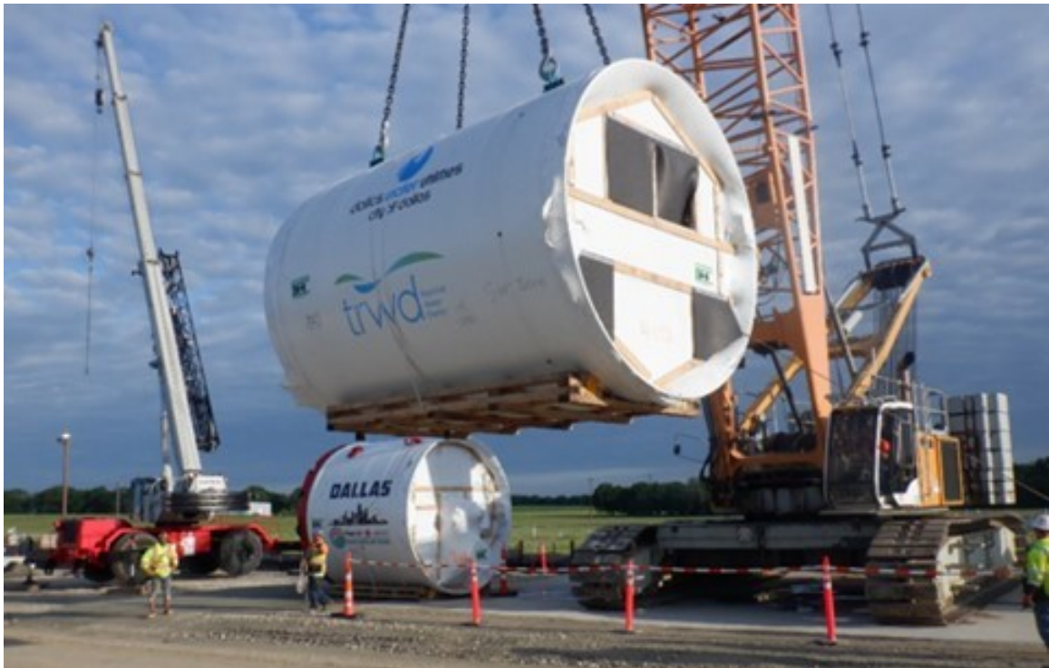
(Tunnel Boring Machine (TBM) operator shield delivery at the pipeline Section 19 Cedar Creek tunnel launch shaft)
