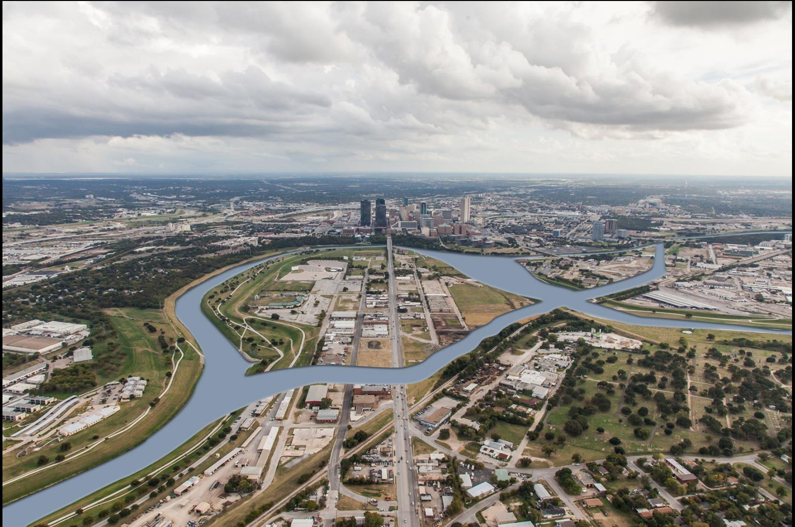
Looking south over Main Street toward downtown
