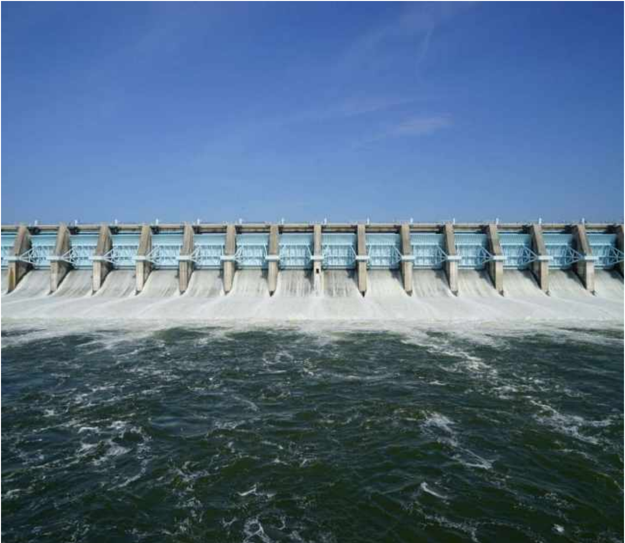
Spillway at Richland Chambers
