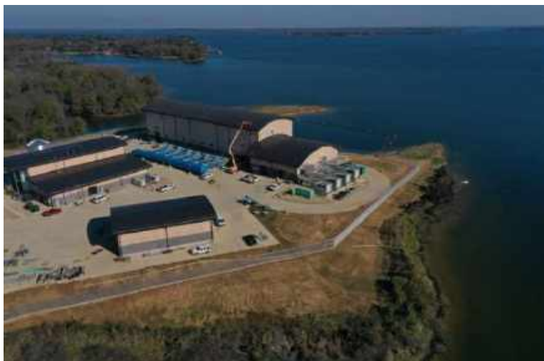
The Joint Cedar Creek (JCC1) pump station came online in fiscal year 2023, increasing pumping capacity and the need for additional chemicals.
