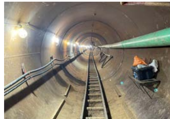
PL19TX US175 Steel Casing Tunnel
