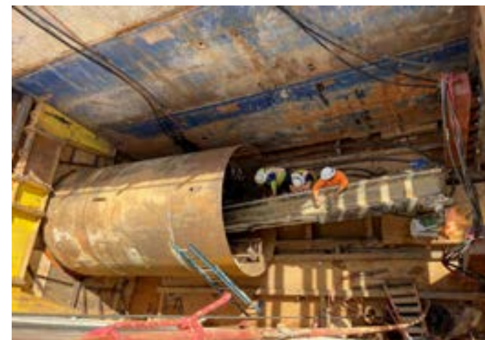
PL19TX Tunnel Excavation at FM1305
