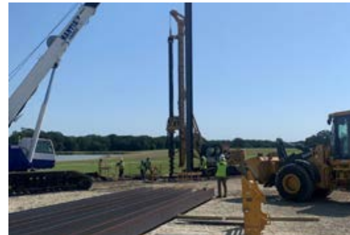
PL19TUN Installing Soldier Piles at Cedar Creek West Portal
