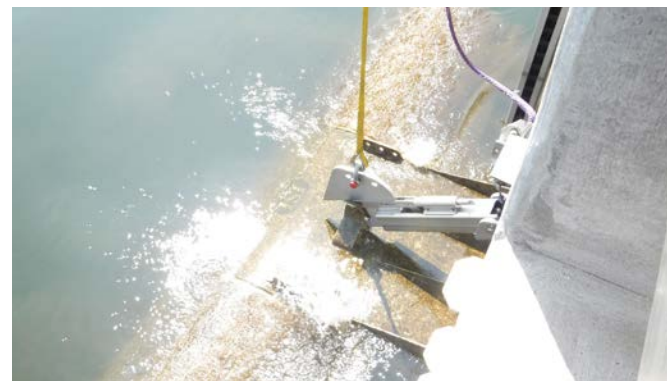
JCC1 Lowering intake tee screens into place
