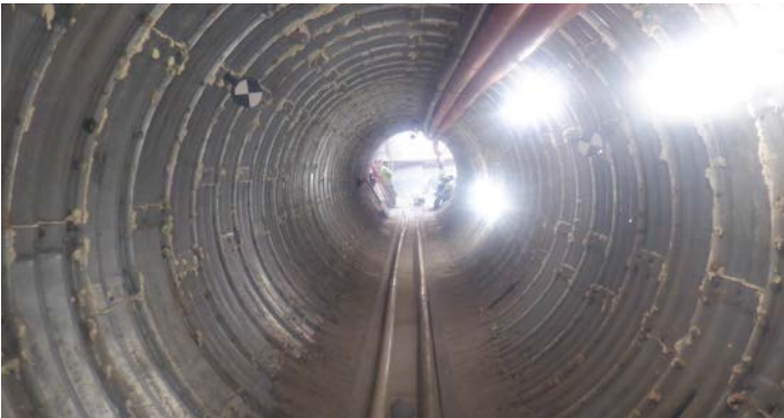
PL19TX Completed tunnel with fiber optic conduits at FM 2636
