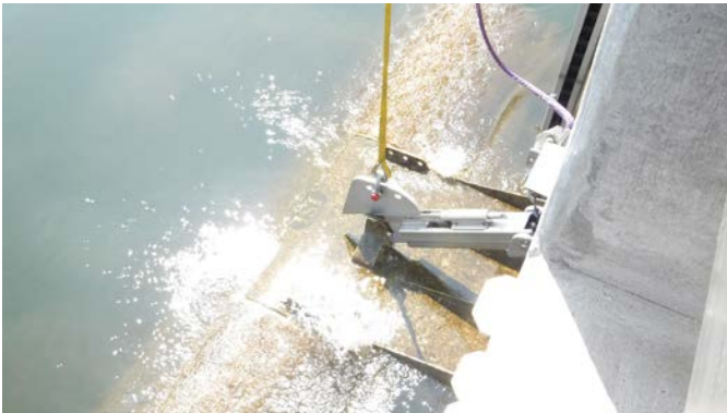
JCC1 Lowering intake tee screens into place
