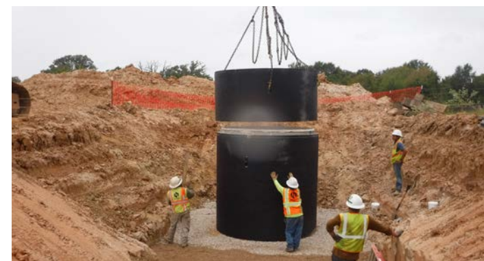
PL19TX Installation of manhole vault at FM 753
