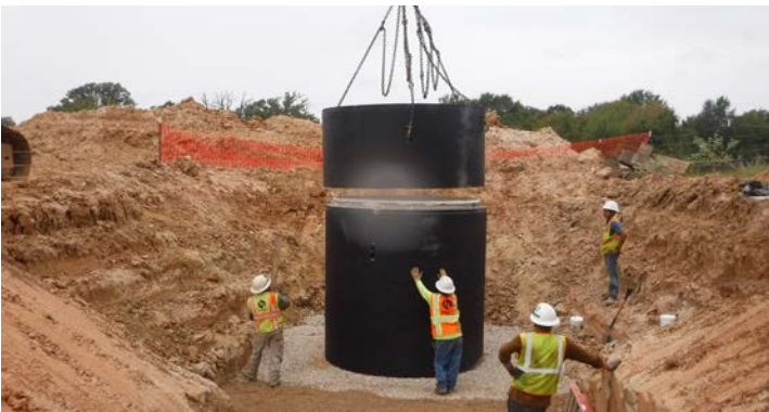
PL19TX Installation of manhole vault at FM 753
