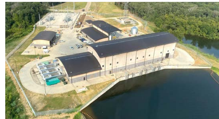
JCC1 Aerial view of Pump Station facility
