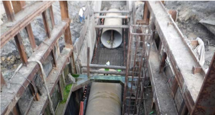
PL17TUN Installing pipe on East Side open cut
