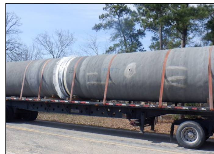
PL19TX Delivering 84-inch tunnel pipe at FM753
