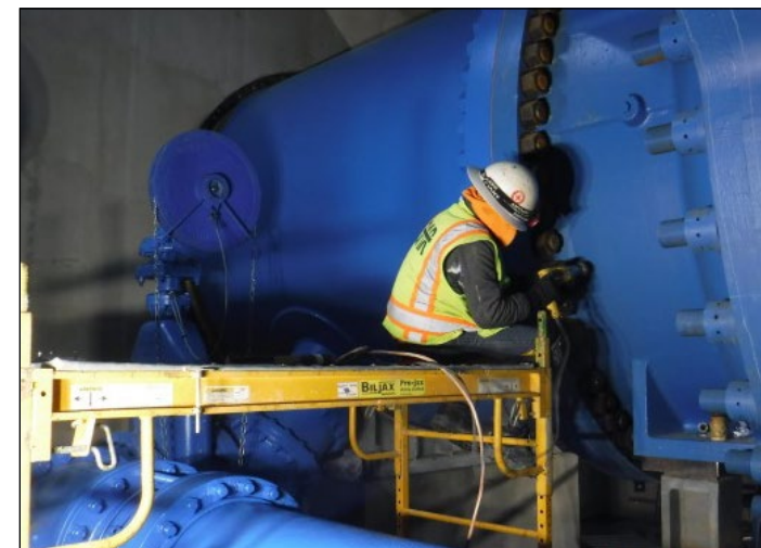
JCC1 Coating 108-inch piping
