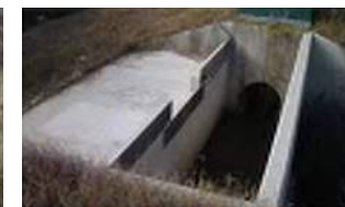
Retention basin, outlet, and inlet structure (Kannan, 2014)
