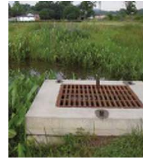
Wet basin multi-stage outlet (SARA Manual, 2013)
