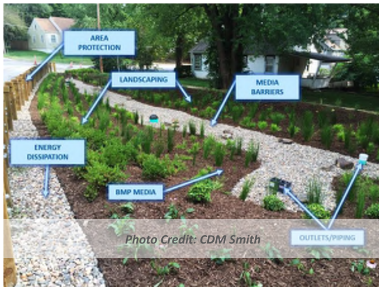
Figure 4.1 Example of Design Components in Bioretention BMP
