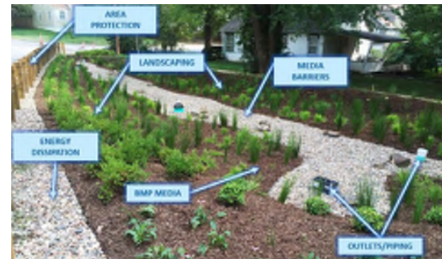
Bioretention Basin with Components Labeled (CDM Smith, 2017)
