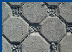
Permeable pavers – aggregate joints (S. Landgren, 2011)
