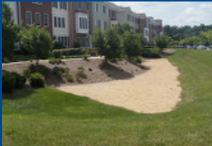
Surface Sand Filter Seneca Best Management Practice. DEP Montgomery County, MD.
