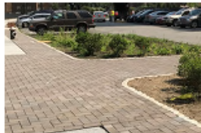
Permeable pavers and rain gardens (Harroch, W., et al., 2017)
