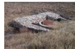
Retention basin, outlet, and inlet structure (Kannan, 2014)
