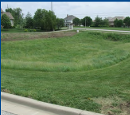
Extended Dry Detention Basin, City of Lenexa, KS
