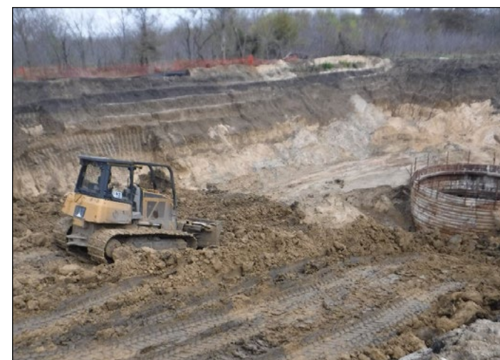
PL17TUN Backfilling west portal shaft
