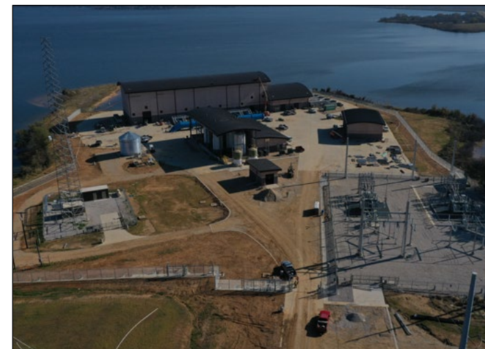
JCC1 December aerial of complete pump station facility
