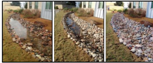
48-hour infiltration of stormwater after a rain event.
