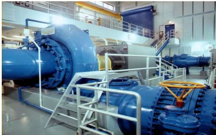
The Hydroelectric Turbine, pictured above, is located at Arlington Outlet and produces electricity which the District sells back to the grid.
