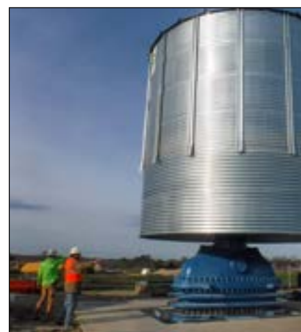
PL1718 Setting silo over 108-inch gate valve at JB2
