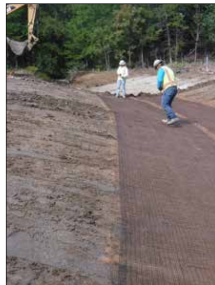
PL1718 Installing turf mat at creek crossing
