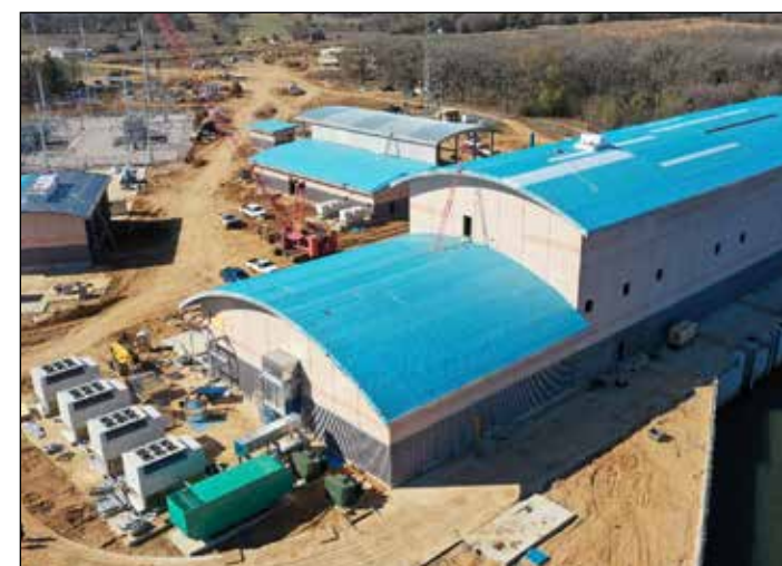
JCC1 Roof installation progress
