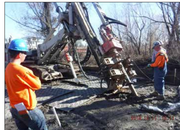
PL17TUN Pre-grouting for soil stabilization
