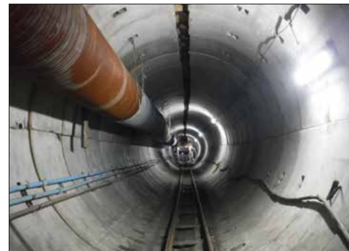
PL17TUN Looking east at tunnel from the access shaft
