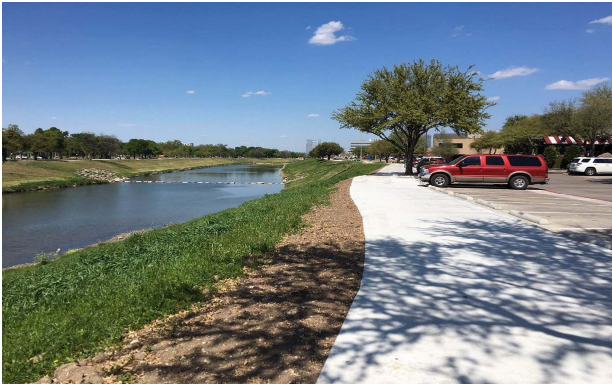
Completed construction of a trail extension on the East Bank at Parkview Ave. This project cost was fully reimbursed from Chisholm Trail Mitigation funds.
