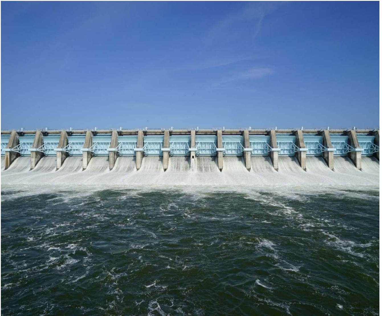
Spillway at Richland Chambers
