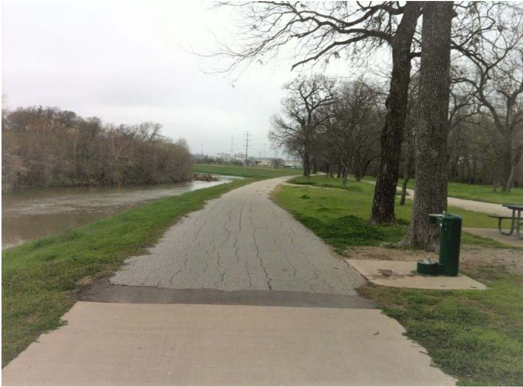
Trail resurfacing enhances the trails for safety and sustainability. Shown here is a resurfacing project that will replace the weathered asphalt.
