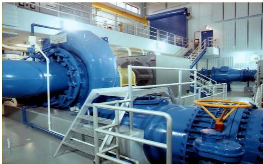
The Hydroelectric Turbine, pictured above, is located at Arlington Outlet and produces electricity which the District sells back to the grid. FY20 income from the sale of power is estimated at $20K.
