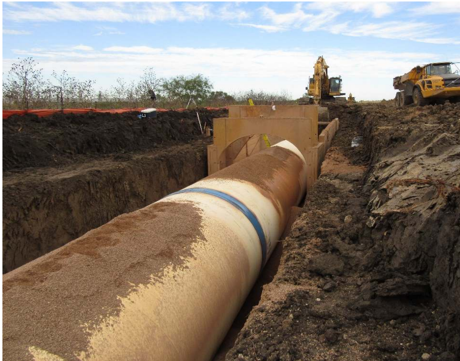
TRWD has a pipe replacement program that utilizes sophisticated technology to identify areas on each pipe segment with the highest potential of failure. Sections of pipe are replaced by the District's crew while demands are low, saving time and valuable dollars. The FY20 Pipeline and Pump station budget includes a $768K budget to replace 14 pipe segments totaling 336 feet.
