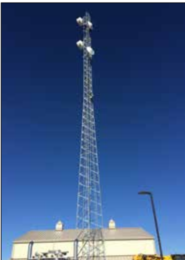
COM01 S5X15 Radio Tower Installation
