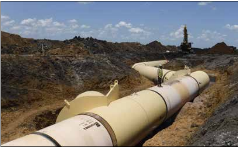
Installation of 108-inch-diameter yard piping at future JB4 Pump Station Site
