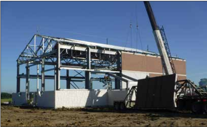
S2X12 Installing pre-cast wall panels at the S2X12 Interconnect facility
