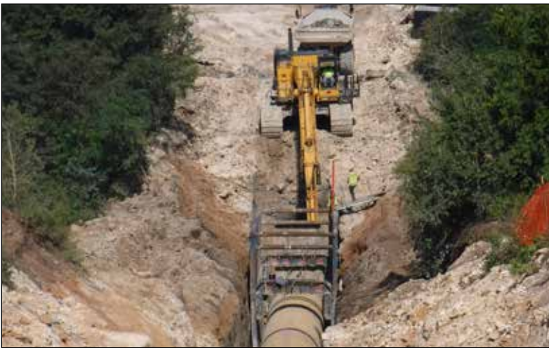
PL14 Installing pipe across Oak Branch Creek Tributary
