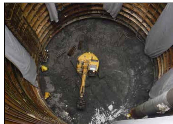
PL17TUN Excavation to deepen tunnel launch shaft
