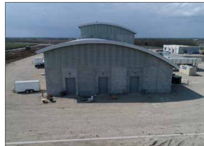
JB3 View from north end of Electrical Room at JB3 Pump Station
