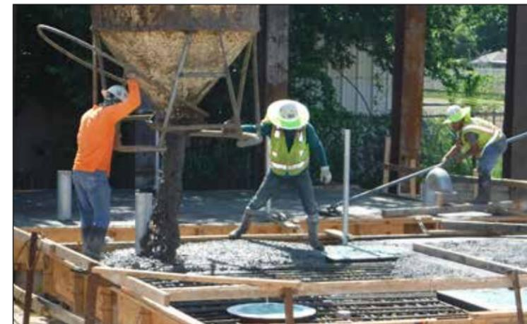
S1X10 Placing concrete for top deck of Venturi Flowmeter Vaults
