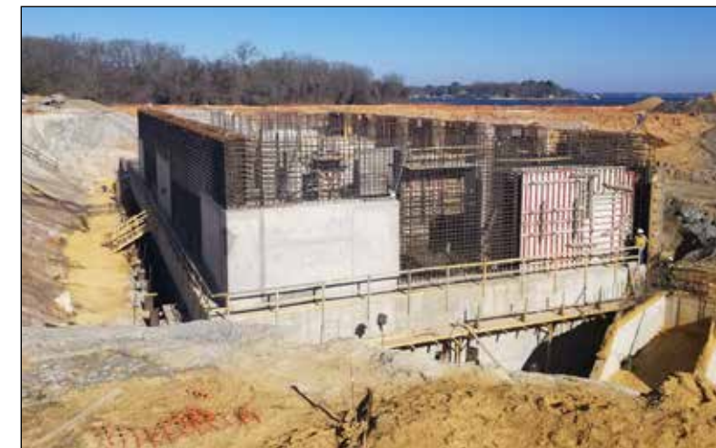
JCC1IN Progress of structural concrete at intake structure
