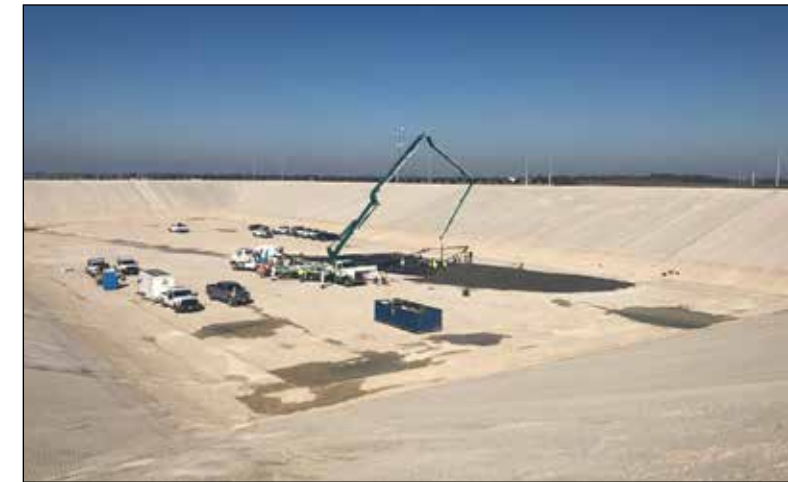
JB3C2 Placing concrete for repair of damage in JB3 Reservoir cell 2
