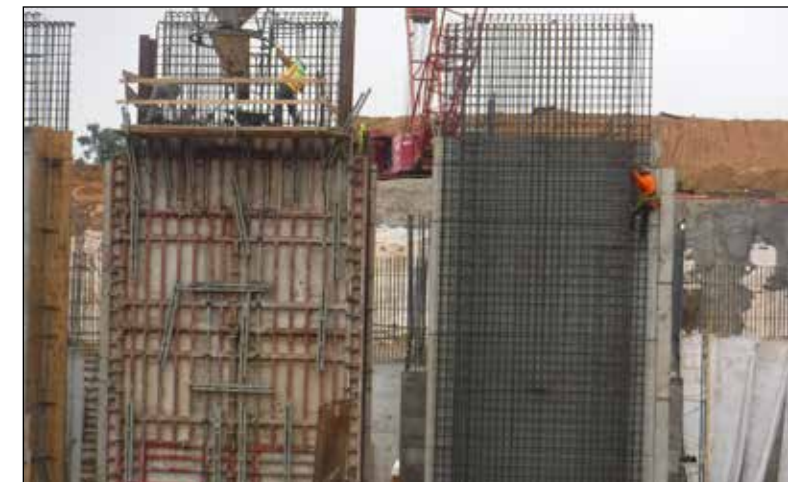
JCC1IN Concrete and rebar placement for front walls
