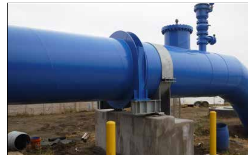
S2X12 Finish coating on 60-inch pipe
