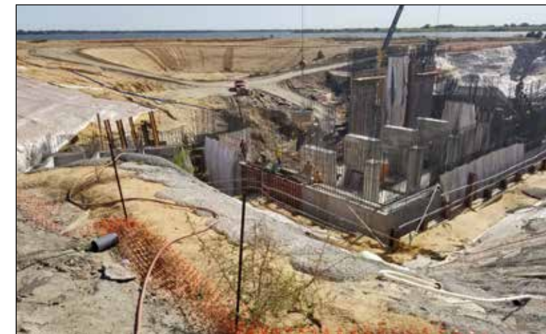
JCC1IN Overview of Intake Structure progress at end of October 2017
