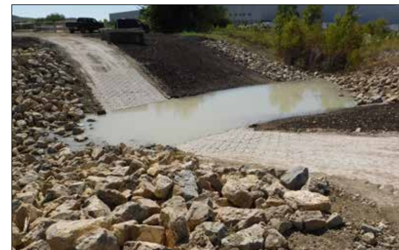
PL1213MBR Cable mat installation in drainage channel near Kemp Ranch Road
