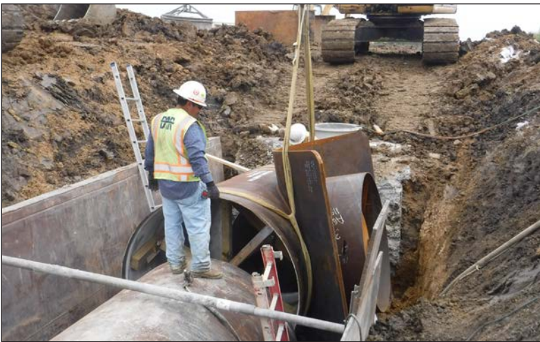
S2x12 Installing 72 x 60 tee in existing Cedar Creek Pipeline for IPL connection
