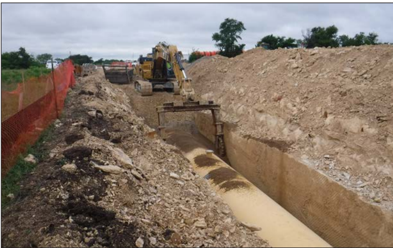
PL14 compacting pipe embedment in rock trench
