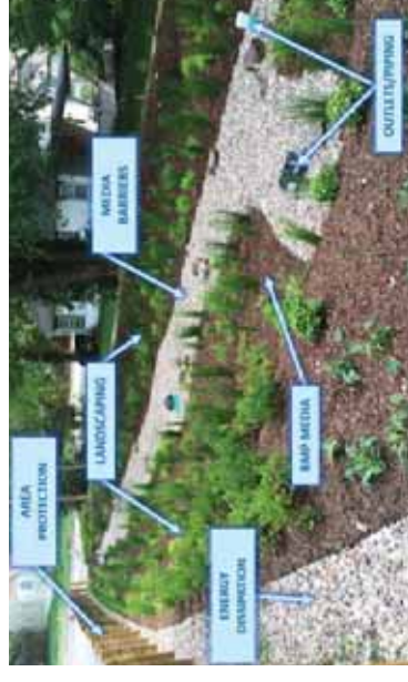
Bioretention Basin with Components Labeled (CDM Smith, 2017)
