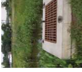
Wet basin multi-stage outlet (SARA Manual, 2013)
