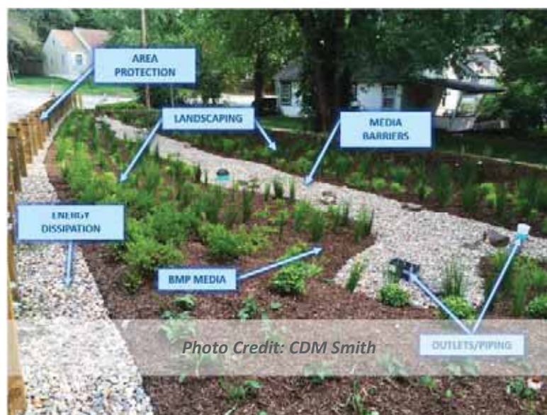
Figure 4.1 Example of Design Components in Bioretention BMP
