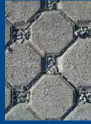
Permeable pavers – aggregate joints (S. Landgren, 2011)
