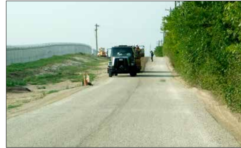
PL1213MBR Making final road repairs to Baucum Road at MBR
