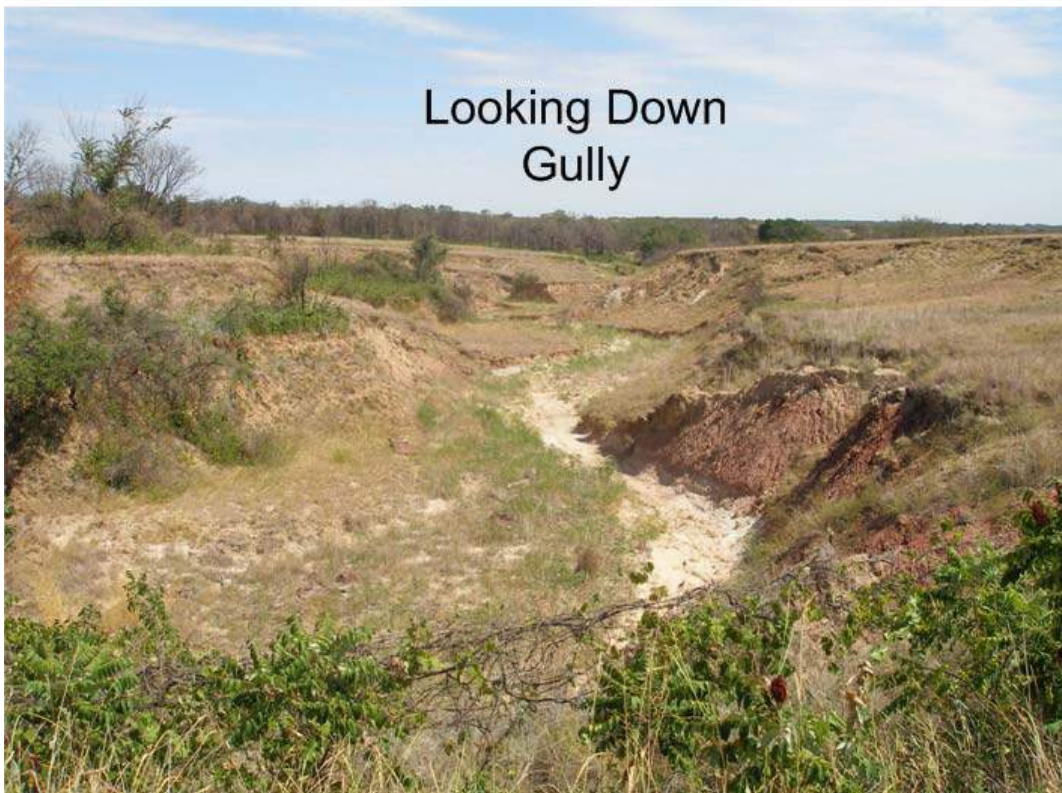
Figure 7. The same gully system (in Figure 6) as seen from the field survey. The gully is temporarily stabilized. Note new floodplain.
