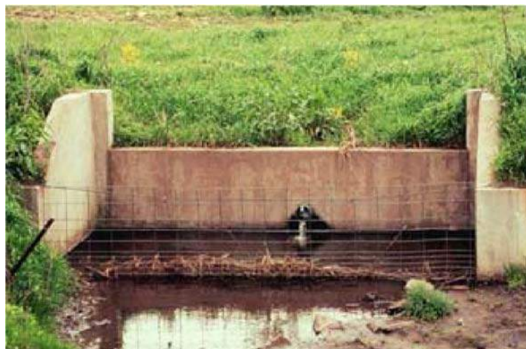
Figure 24. Graded Stabilization Structure
