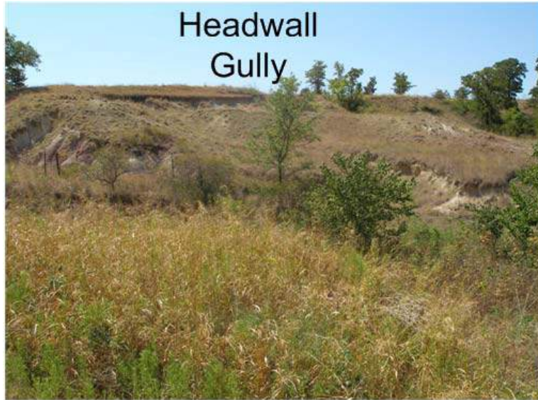
Gully Erosion RD Location
