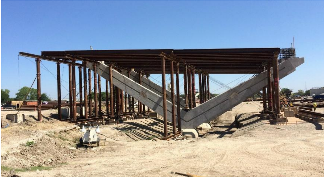
(White Settlement V-Piers for bridges under construction)
