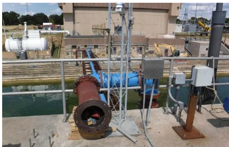
(12" Flash mix line and chemical lines across the bridge to the Richland Chambers Lake Pump Station intake structure)
