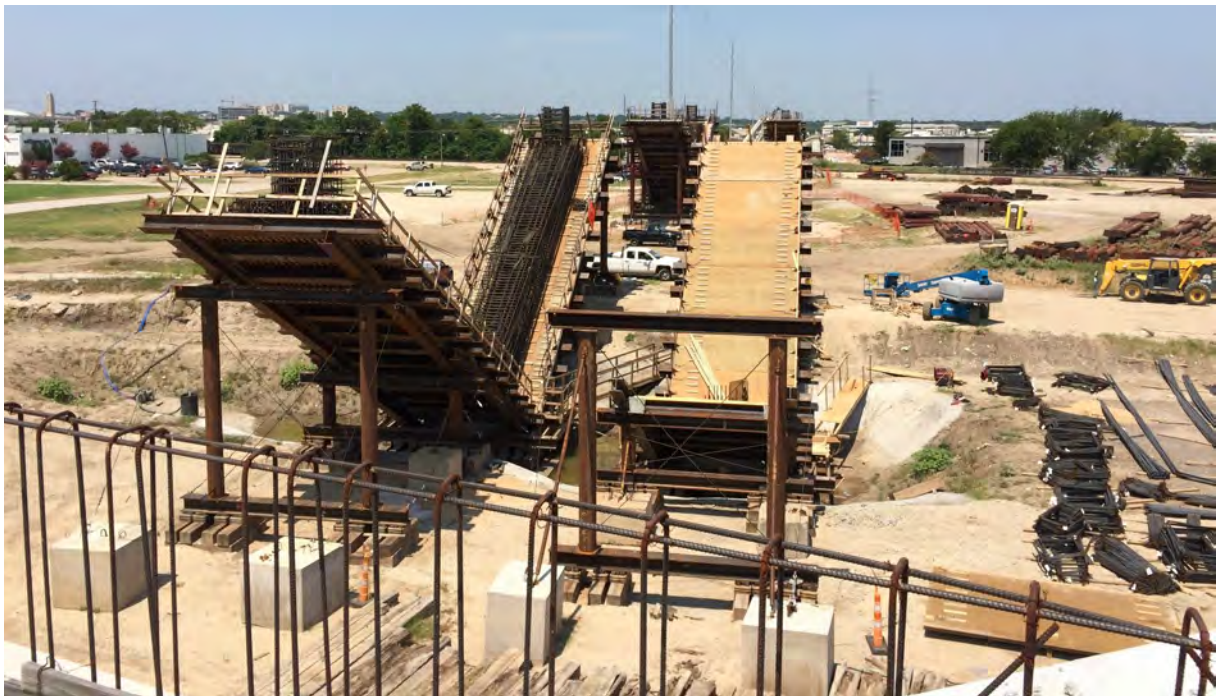
(V-Piers for Panther Island Bridges under construction)
