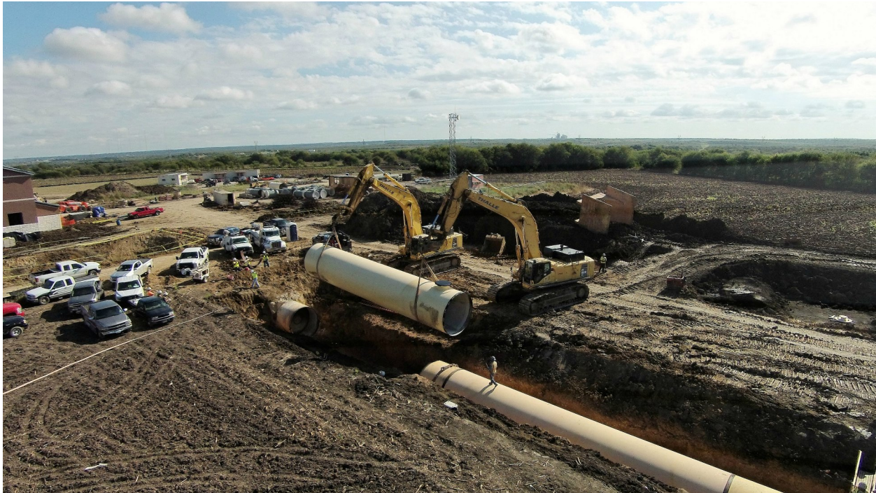
(Photo of installation of 108 inch pipe at Midlothian Balancing Reservoir )
