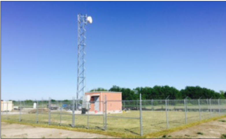
COM01 Microwave tower at S2X12 site
