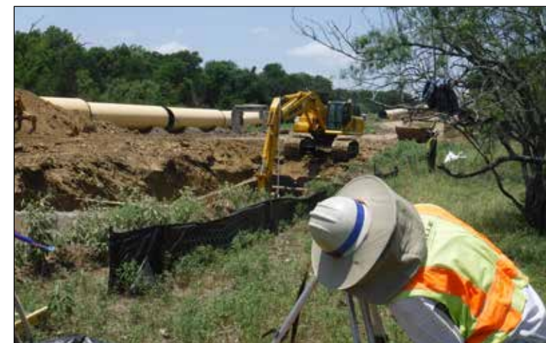
PL1718 Verifying top of pipe elevation
