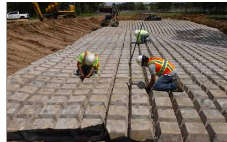
PL1011 Installing cable mat low water crossing
