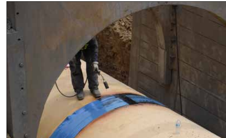
PL1718 PD Installing heat-shrink joint wrapper on 108-inch pipe
