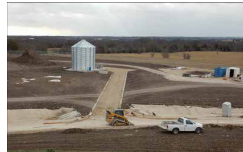
PL1213MBR Site Roads and 108-inch Gate Valve Silo
