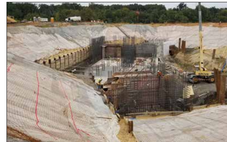
JCC1IN overview of the intake structure
