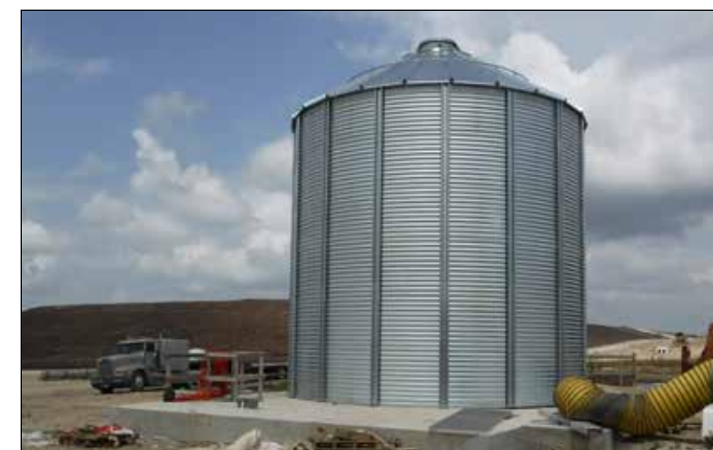
PL1213MBR Silo over gate valve on bypass line at MBR
