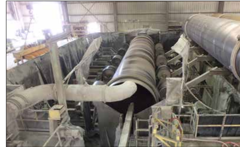
PL1718 Spinning cement mortar lining in 108-inch pipe
