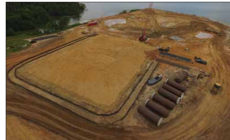
JCC1IN Aerial view of soil stockpile for pre-settlement of future chemical facility
