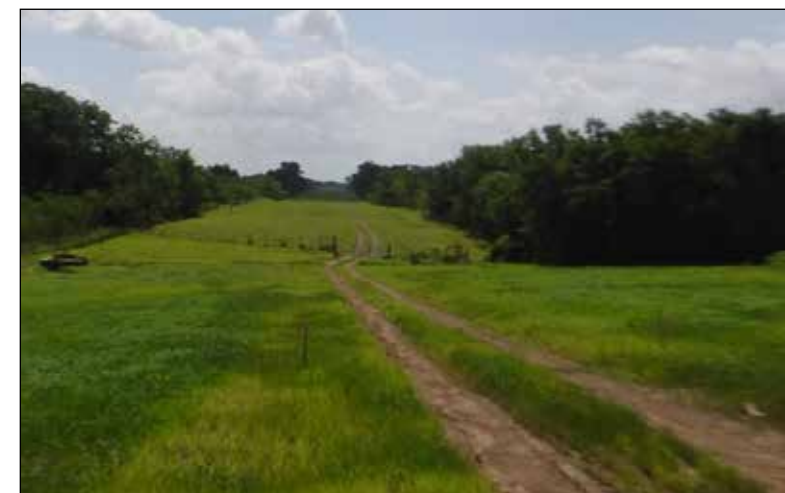
PL152 Progress of ROW restoration and grassing
